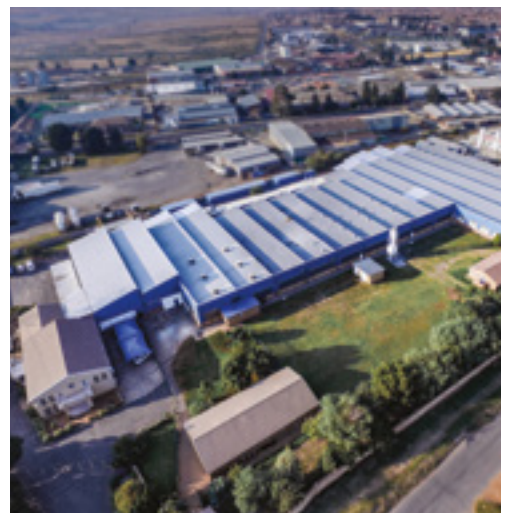
Grinding Techniques headquarters in Chamdor (Krugersdorp)
