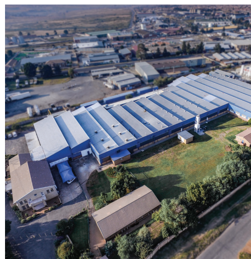
Grinding Techniques headquarters in Chamdor (Krugersdorp)
